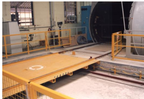
This traversing platform manufactured for Aerostructures takes product to and from their autoclaves
